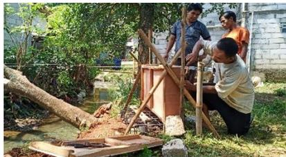
Gambar 11. Pemasangan Bekisting Abutmen
