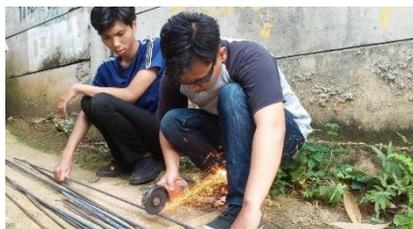
Gambar 7. Proses Pemotongan Tulangan Abutmen
